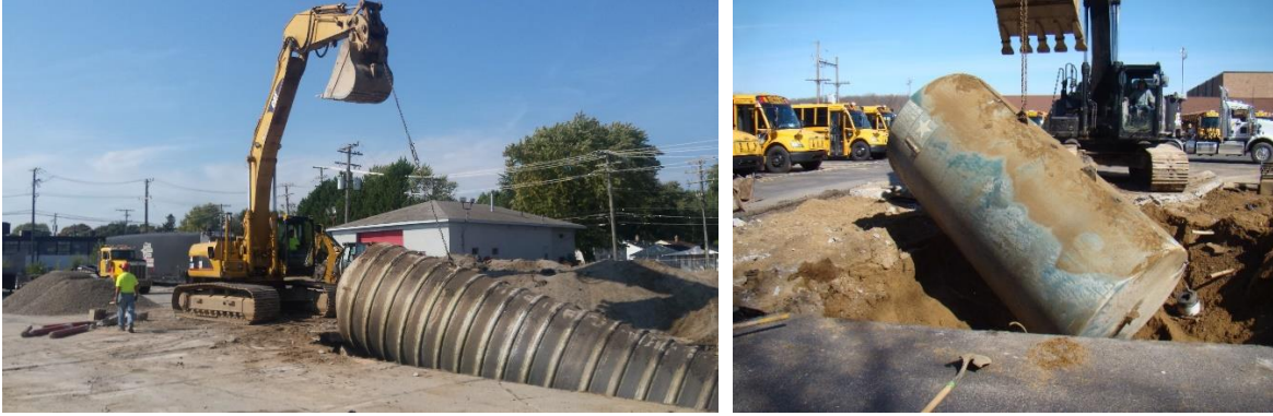
Images (left and right): Removal of gasoline USTs.
